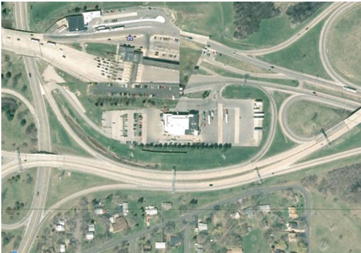
Figure U.9. Bonner Bridge POE
