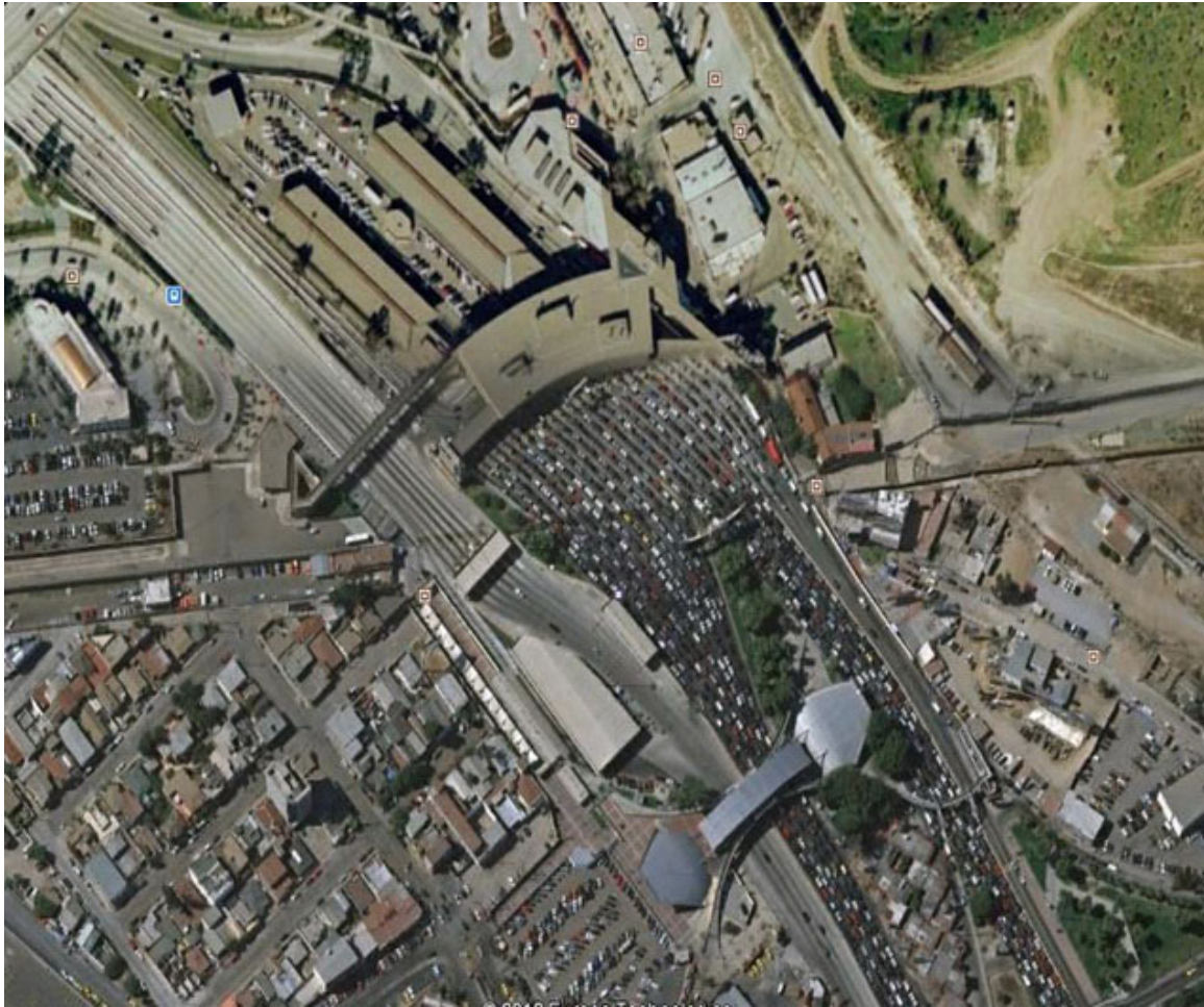
Figure U.6. Tower Beach POE
