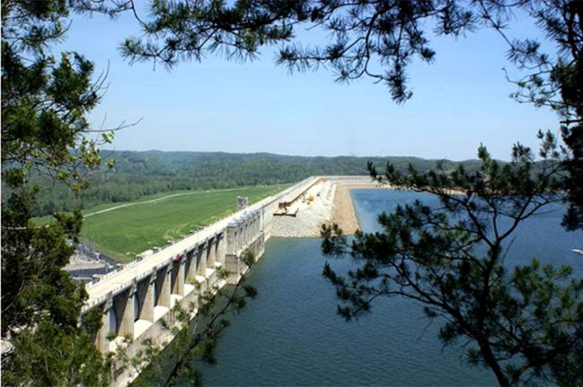
Figure J.18. East Lake Dam
